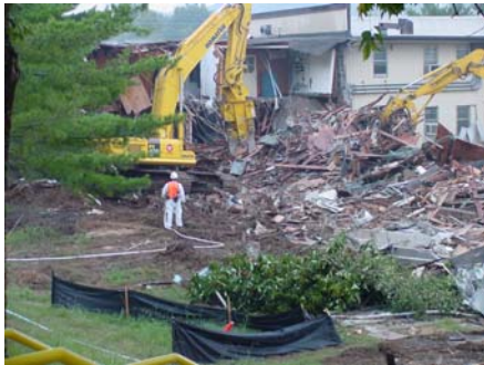
Demolition of ORNL Building 1000
