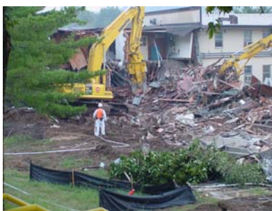
Demolition of ORNL Bldg. 1000
